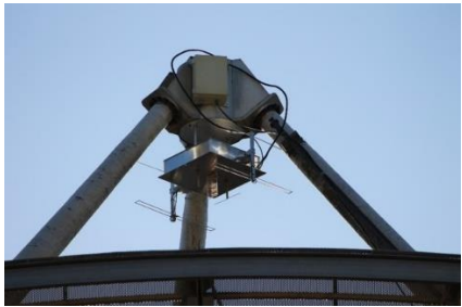
Figure 2: Feed Installed on dish
