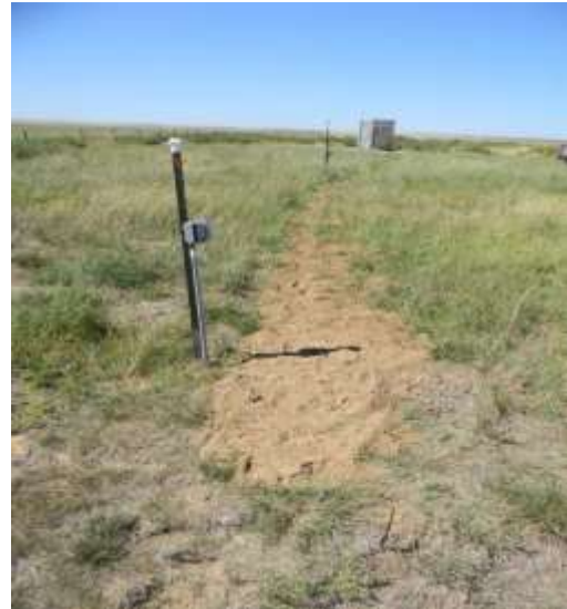
Figure 5 The RV Power Hookups wiring trench was dug and buried.
