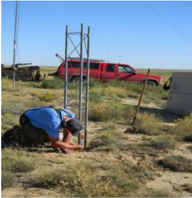
Figure 13 Ed Corn installing the tower base section
