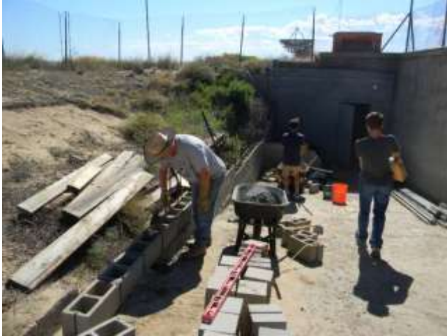
Figure 11 Dave, Alex and Hans building the ramp wall
