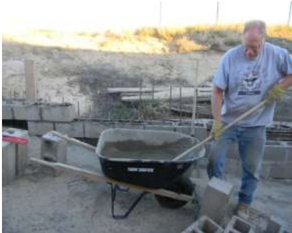
Figure 10 Dave Molter working on his ramp wall replacement project
