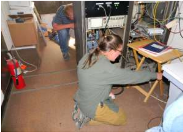
Figure 8 Francis Royo tracing down and labeling power outlets
