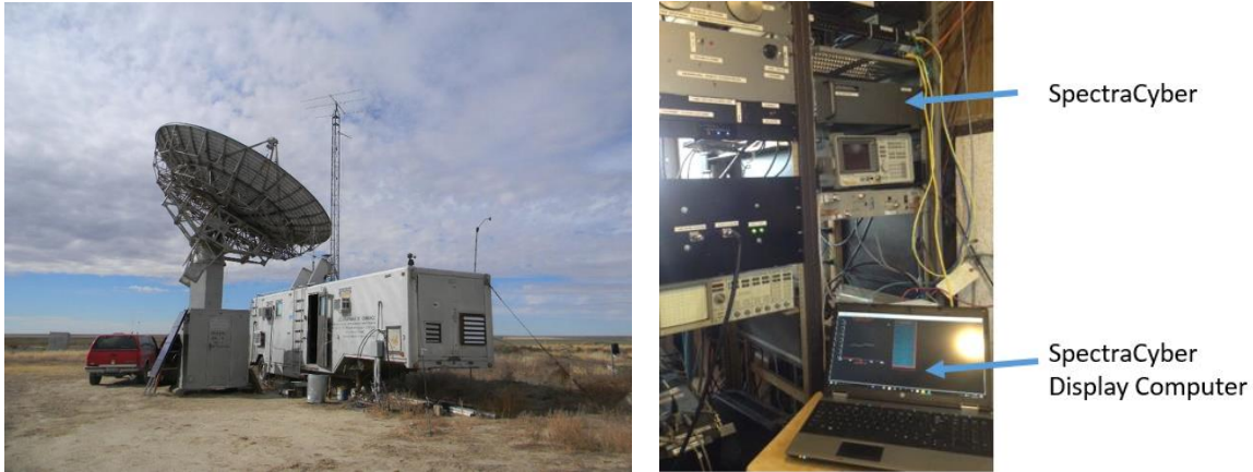
Figure 3: Communications Trailer and Equipment Rack
