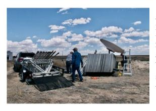
Next came the petals and struts that Rick K0GD towed. Ray and RC dragged more railroad ties over next to a small dish antenna and Rick, Ray, RC, Vlad and Bill began the job of removing the petals and stacking them on their side using a ladder to keep them upright during stacking.
